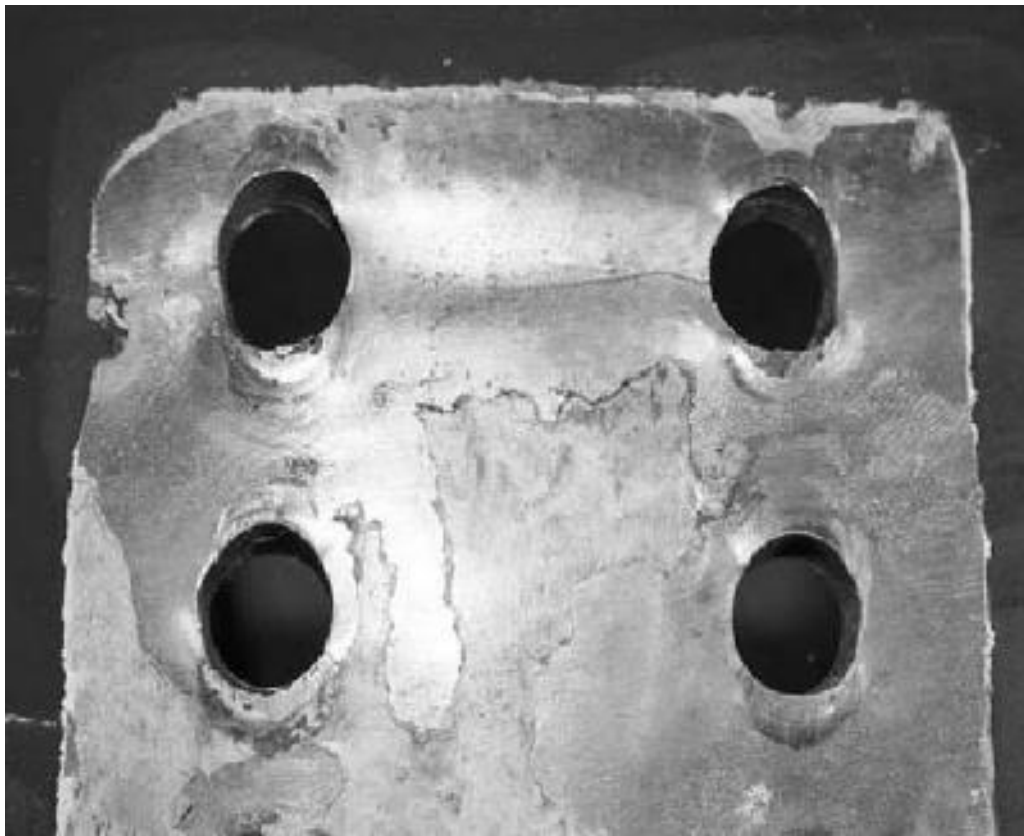
Figure 10.16 Bearing failure of plates
